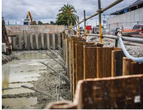
Figure 1: Sheet Pile and Anchor
