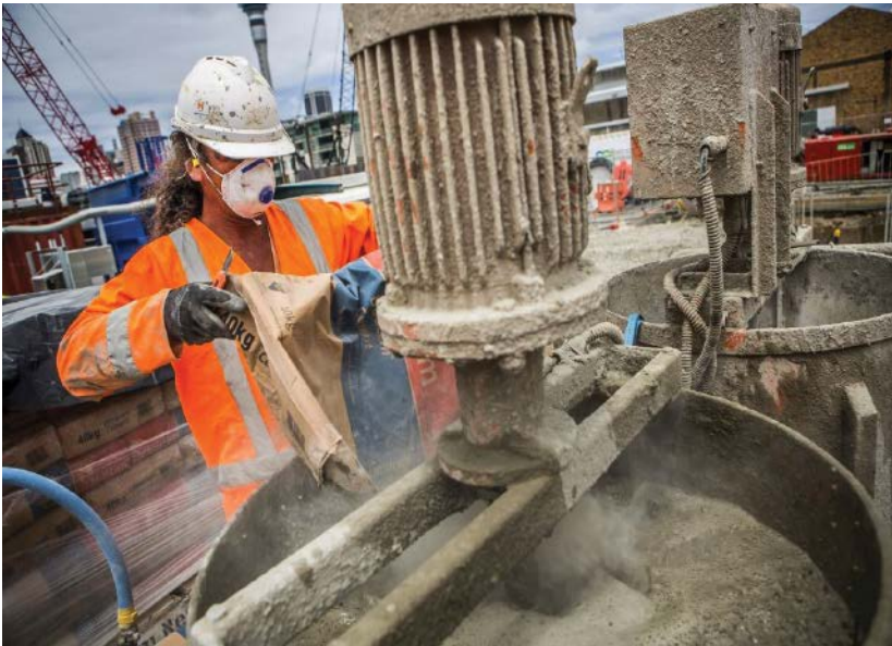
Figure 7: Grouting Station
