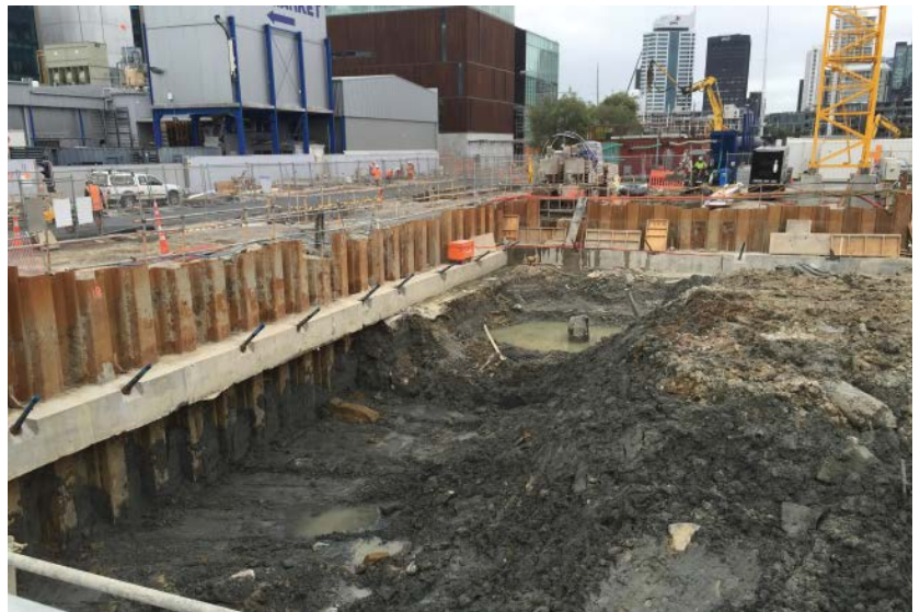
Figure 2: Concrete Waler Beam
