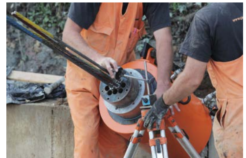
Figure 8: Typical Stressing Set Up
