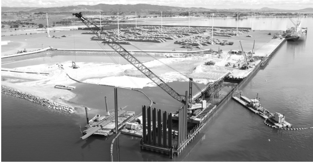
Figure 2: Construction of twin king pile wall at Berth 3
