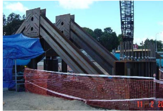
Figure 4: Test pile reaction frame
