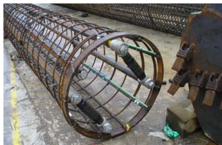
Figure 2b: Pile spoil grouting pipe work
