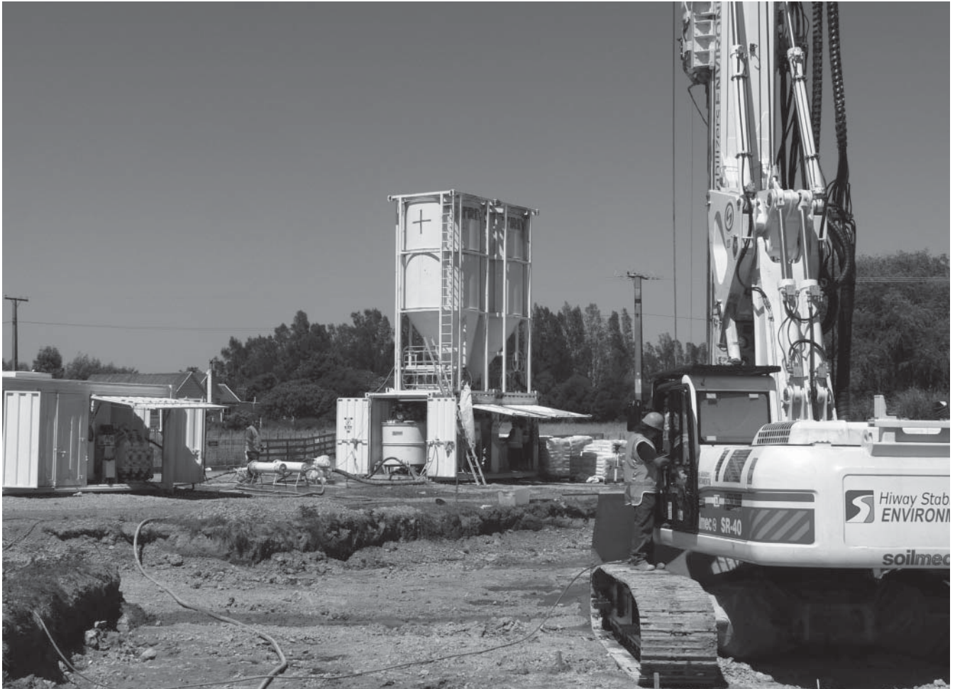
Figure 2a: Turbojet plant – Grout batching plant and high pressure pump
