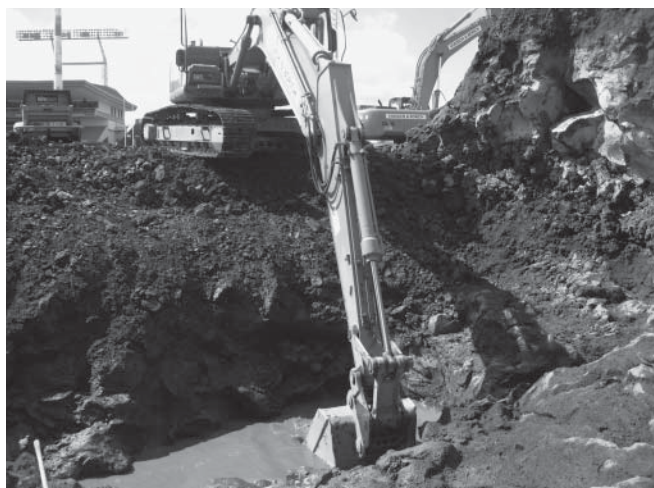
Above left and right: A deep, vertical hollow within the foundation excavation filled with water. This was pumped out and cleaned prior to the construction of the foundation itself.
