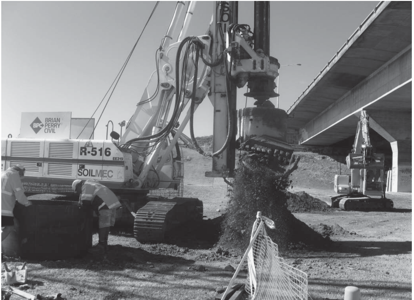
Figure 2: Drilling 1800mm diameter MHX Test Pile
