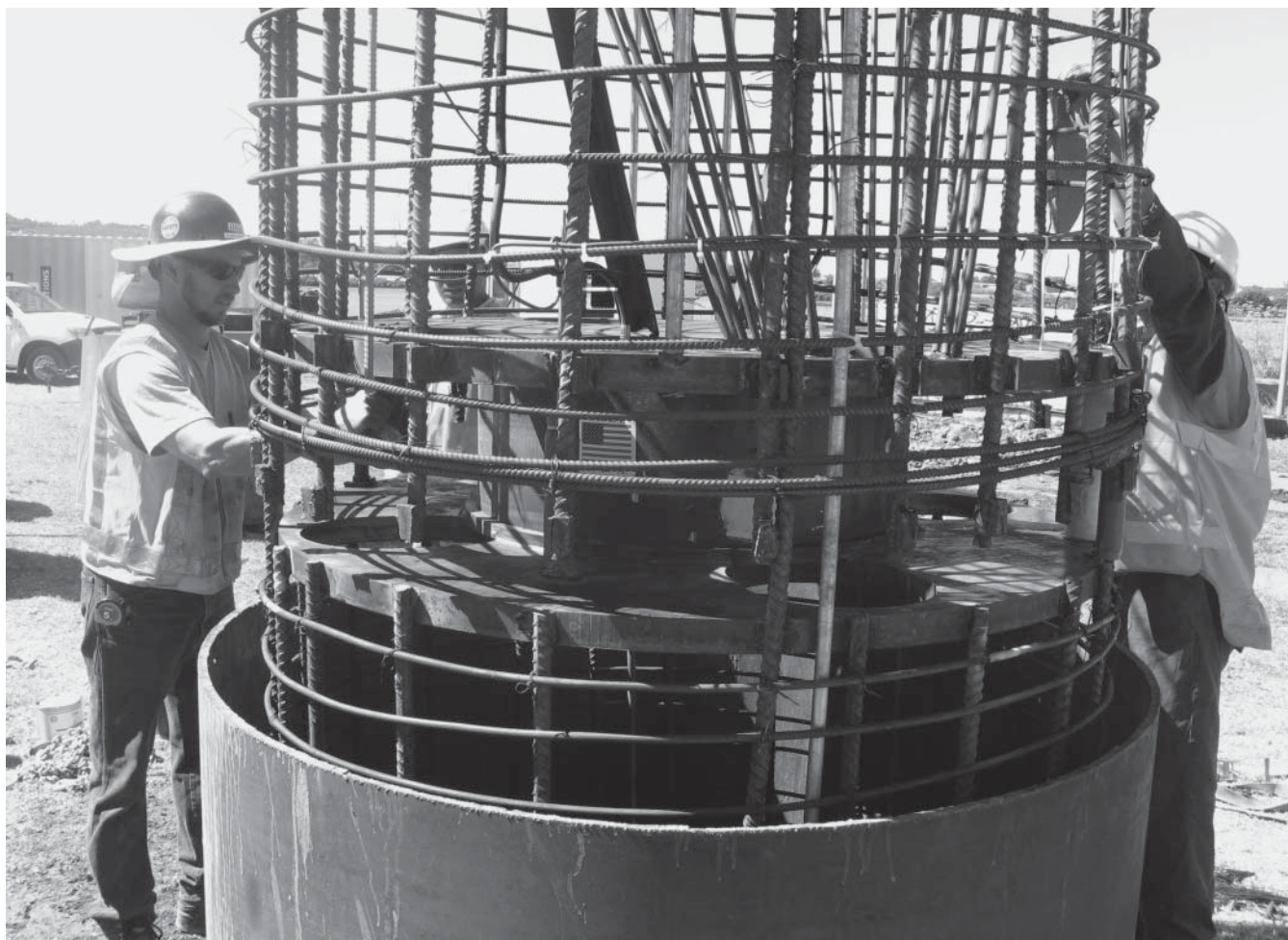
Figure 3: Installation of O-Cell within reinforcement cage of test pile.
