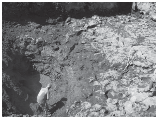
Above left and right: A deep, vertical hollow within the foundation excavation filled with water. This was pumped out and cleaned prior to the construction of the foundation itself.
