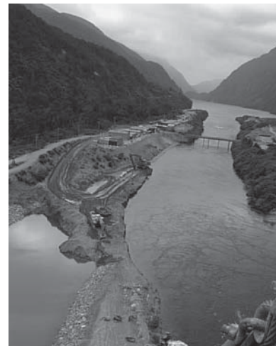
Below: Digging the new channel for the second tail race, Manapouri
