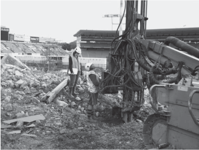
Above left: Proof drilling at foundation excavations Right: Finished foundation excavation
