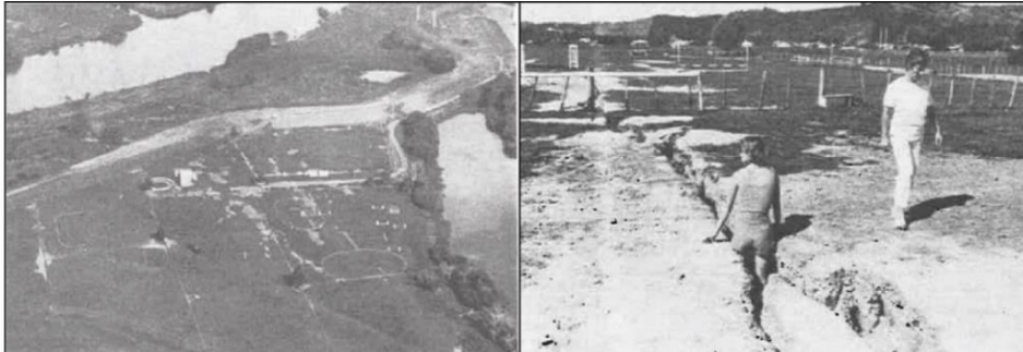
Figure 3: Historical photographs outlining the occurrence of liquefaction in Whakatane following the 1987 Edgecumbe earthquake (Collated from Christensen (1995)).
