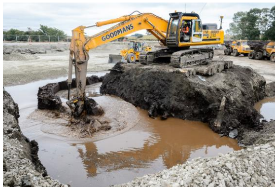
Figure 2 Excavate and replace at the Paetawa Bridge Site.
