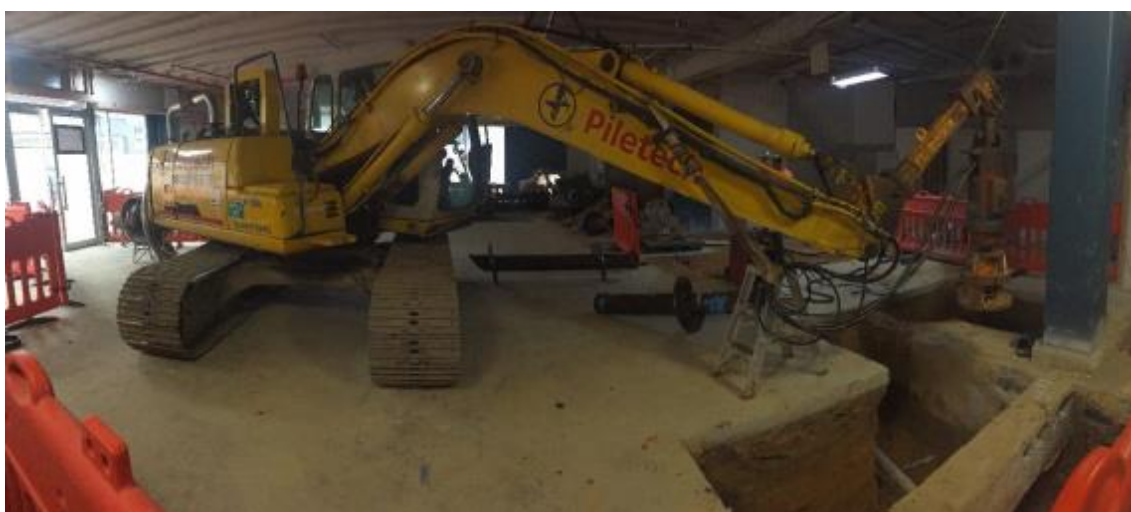
Figure 6: Stage 1 installation of screw piles (Lavin et al, 2016)
