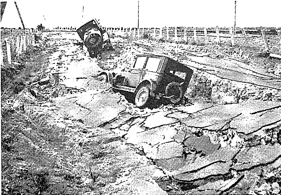
Figure 2. Lateral Spreading of Road Embankment in Napier Earthquake, 1931
