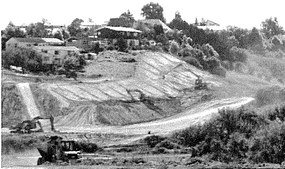
Figure 2. Overview of J3 Cut
