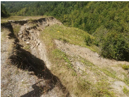
Slope failures in Bozkurt district due to heavy rain
