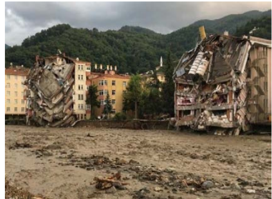
Figure 3. Dragged and crushed vehicles and woods in Bozkurt district and collapsed buildings due to toe erosion during flooding in Ezine stream bed
