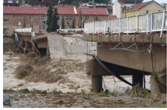
Figure 2. Flooding of Ezine stream in Bozkurt district and collapsed bridge on constructed Ezine stream bed
