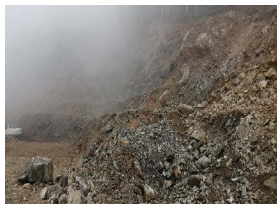
Slope failures in Bozkurt district due to heavy rain
