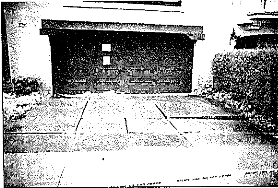
Figure 6 Building settlement as a result of sand liquefaction.
