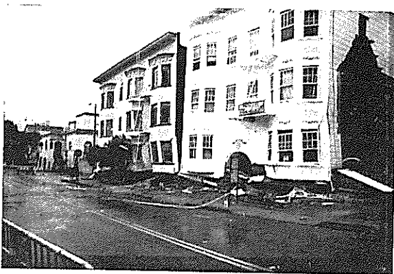
Figure 4 Structure collapse as a result of ground shaking.
