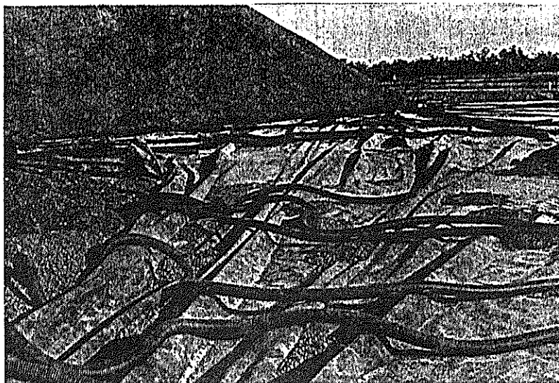
Figure 4. Case Study Liner Deformation
