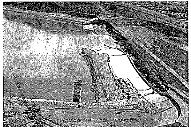
Figure 1 – Damage to the Lower San Fernando Dam. (Steinbrugge Collection, EERC, UC Berkeley)
