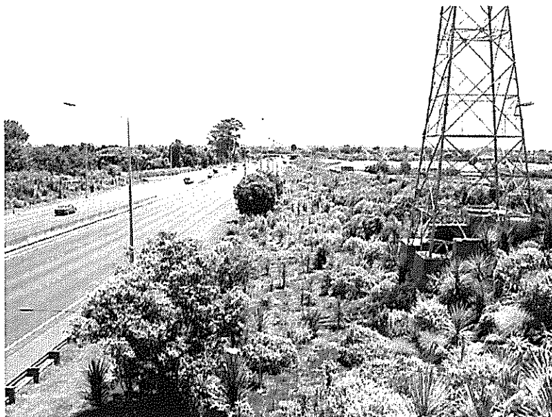
Figure 7. Stable Embankment with Fully Grown Vegetation – ETCART Project
