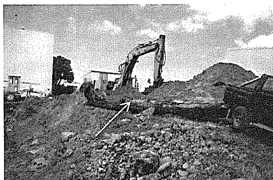
Figure 7. Photograph of the tuff and basalt boundary (dashed line) beneath the Accommodation block. The totara log removed from the tuff (arrow) was carbon dated at 23,480 \pm 180 BP.
