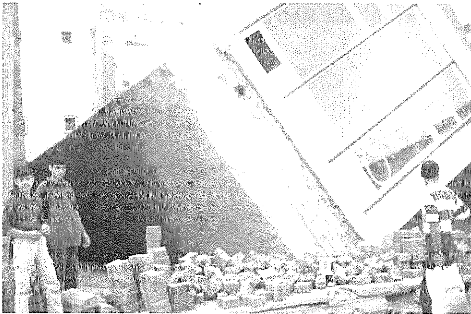
Figure 1. Overturned Building in Adapazzari
