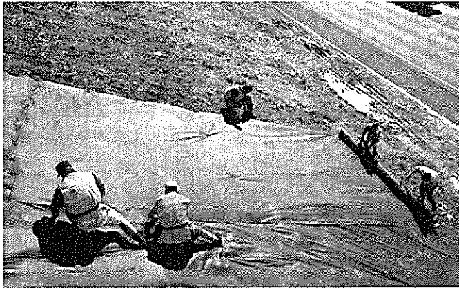
Figure 1. Installation of Geotextile on Embankments
