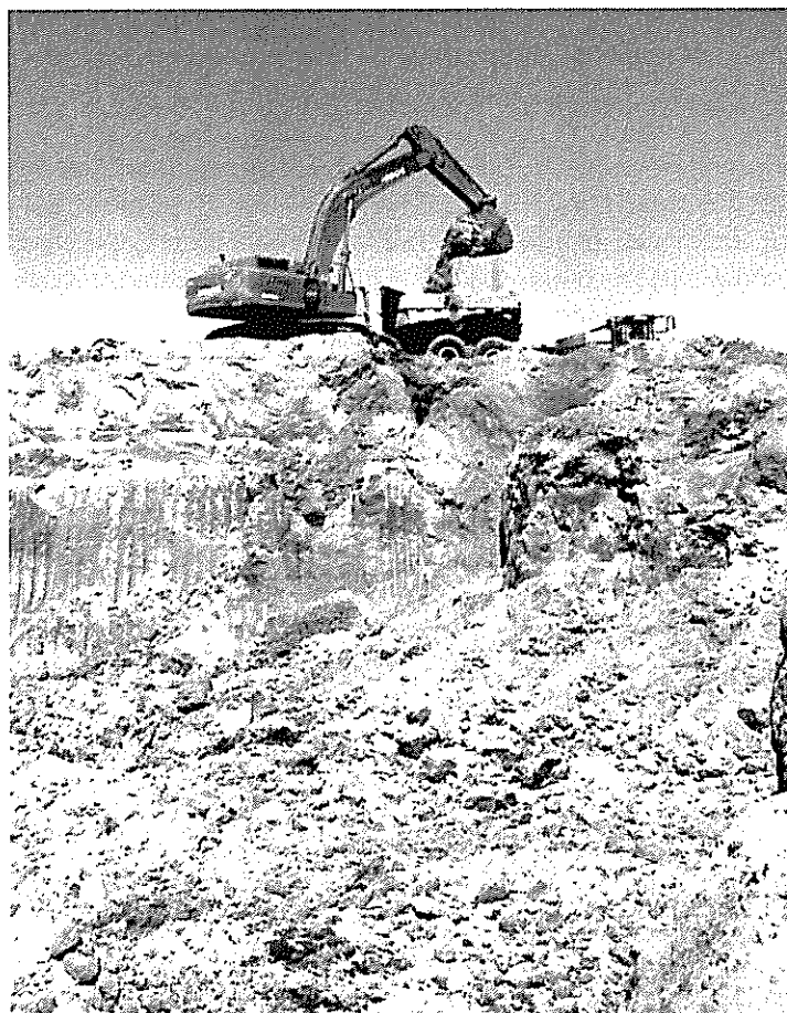
Figure 8. Single Large Excavation Lift
