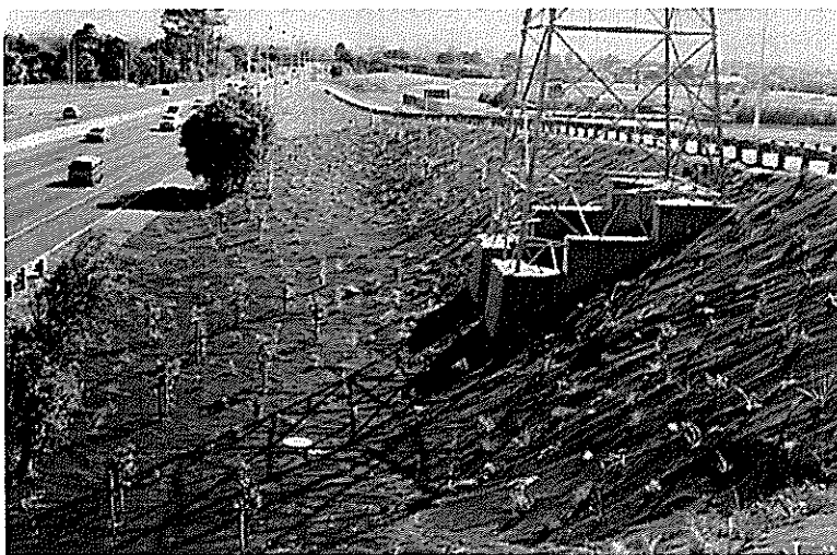
Figure 6. Stable Embankment without Vegetation – ETCART Project
