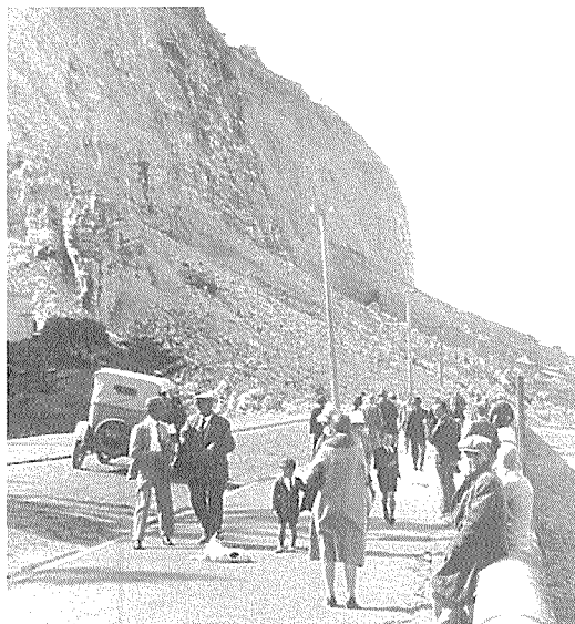
Figure 2. 1931 landslip blocking road to port © Napier City Council
