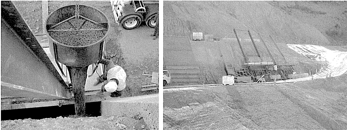
Figure 5: “No fines” concrete installation
