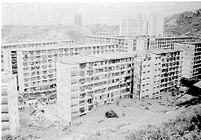
Figure 1: Sau Mau Ping Landslide, 18 June 1972. Ground floors of the buildings were filled by debris, resulting in 71 deaths
