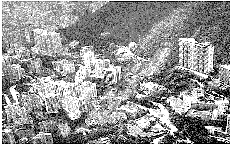
Figure 2: Po Shan Road Landslide, 18 June 1972. A four-storey building and a 15-storey apartment block were demolished during the landslide, resulting in 67 deaths
