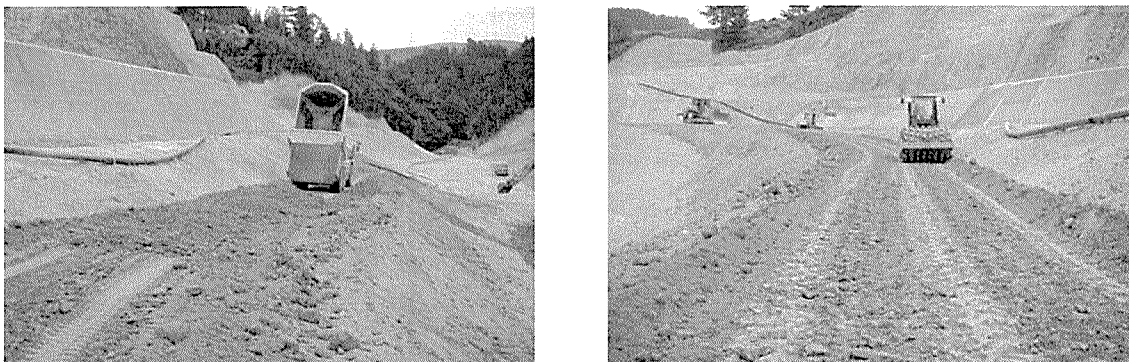
Figure 4: Low permeability compacted clay soil installation
