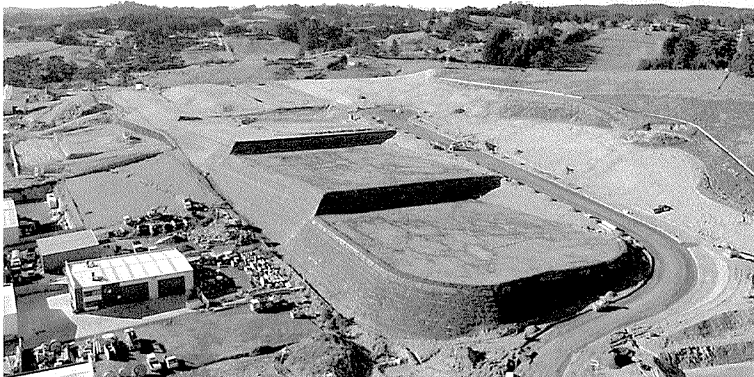
Figure 2: Reinforced Soil Slope during construction.
