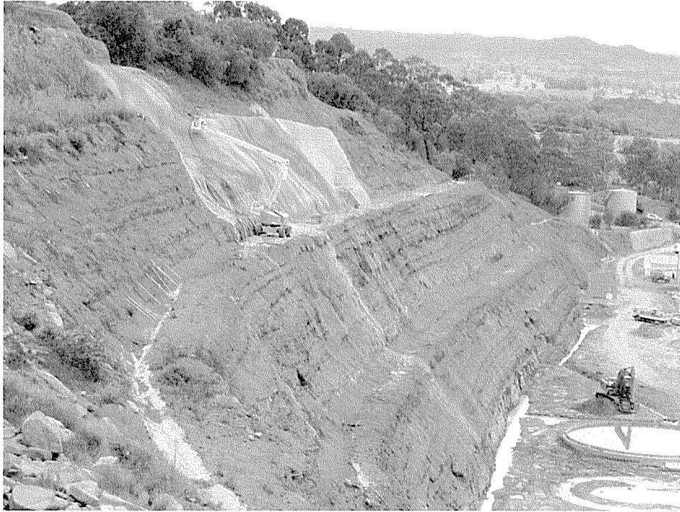
Figure 2: Stabilisation works in progress
