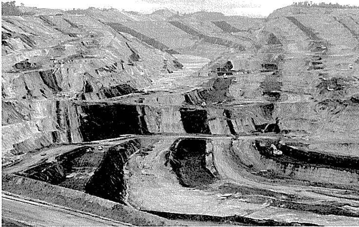
Figure 1: View of part of the Tutupan Coal Mine.
