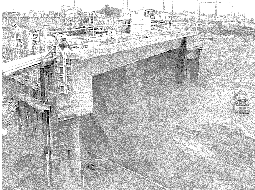
Figure 2: Showing the interbedded sands and silts of the Hinuera Formation
