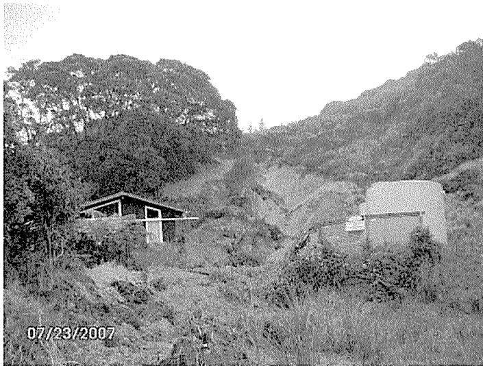
Figure 4: Looking west at headscarp of landslide
