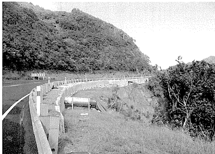
Figure 6: Photograph of the Completed Wall
