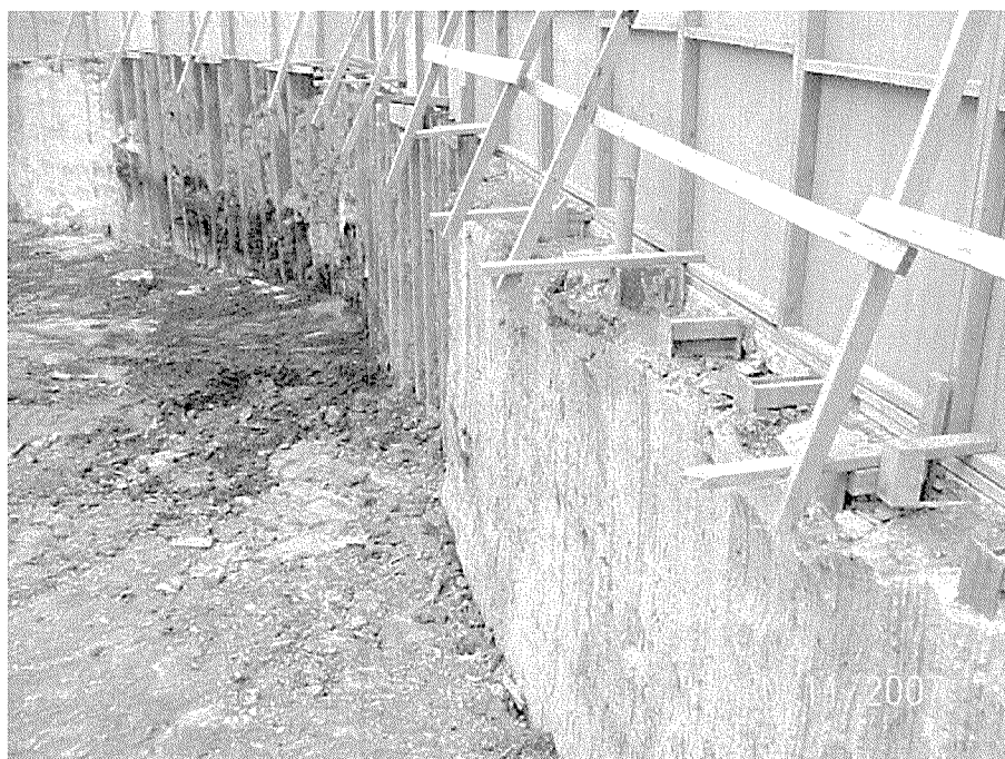
Figure 4: Sheet pile and CSM wall at Fanshawe Street, Auckland
