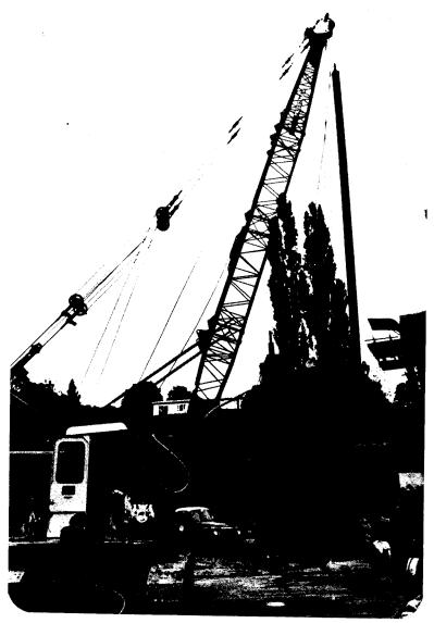
Hamilton Boundary Rd Bridge 2000 mm diam. bored piles 40 metres deep, raked 1 in 10 belled to 4000 mm diam.
