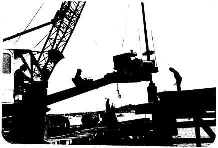
Marine Steel Slipway for 1000 tonne ships. 750 mm diam. piles drilled 8.5 metres from staging centre.
