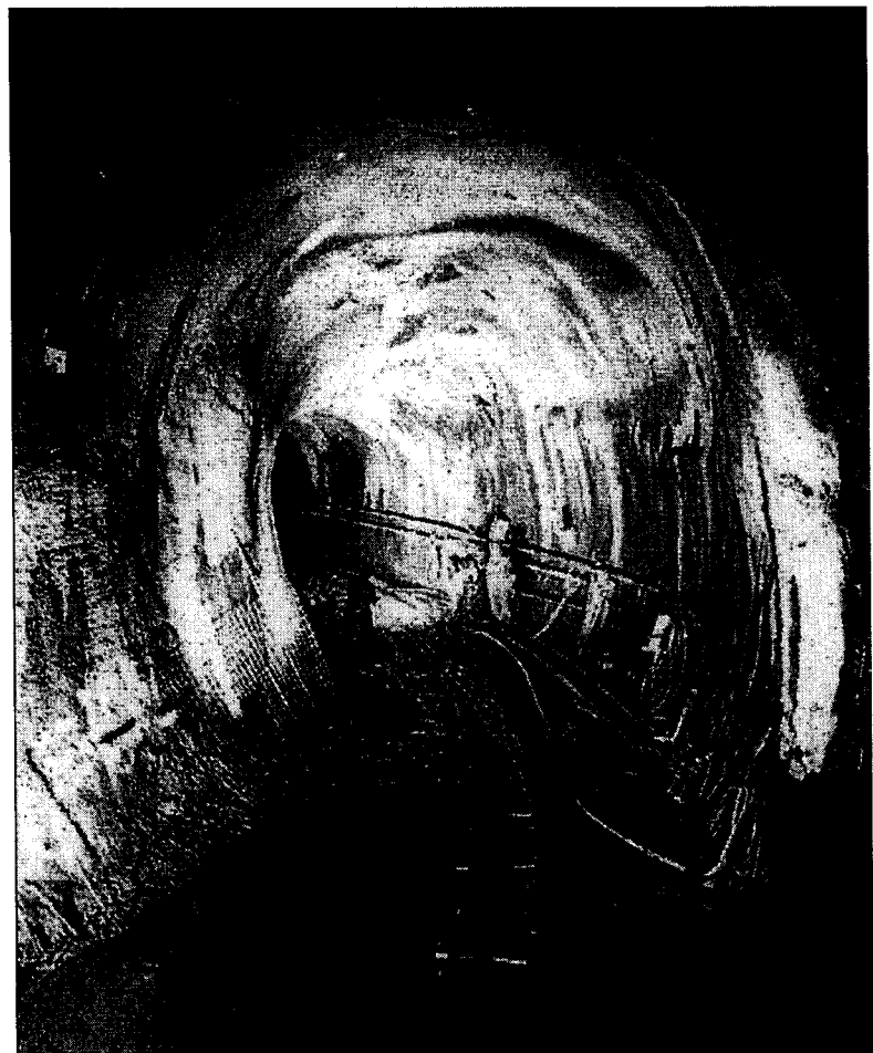
First contact – TBM hole through from Penrose to Newmarket
