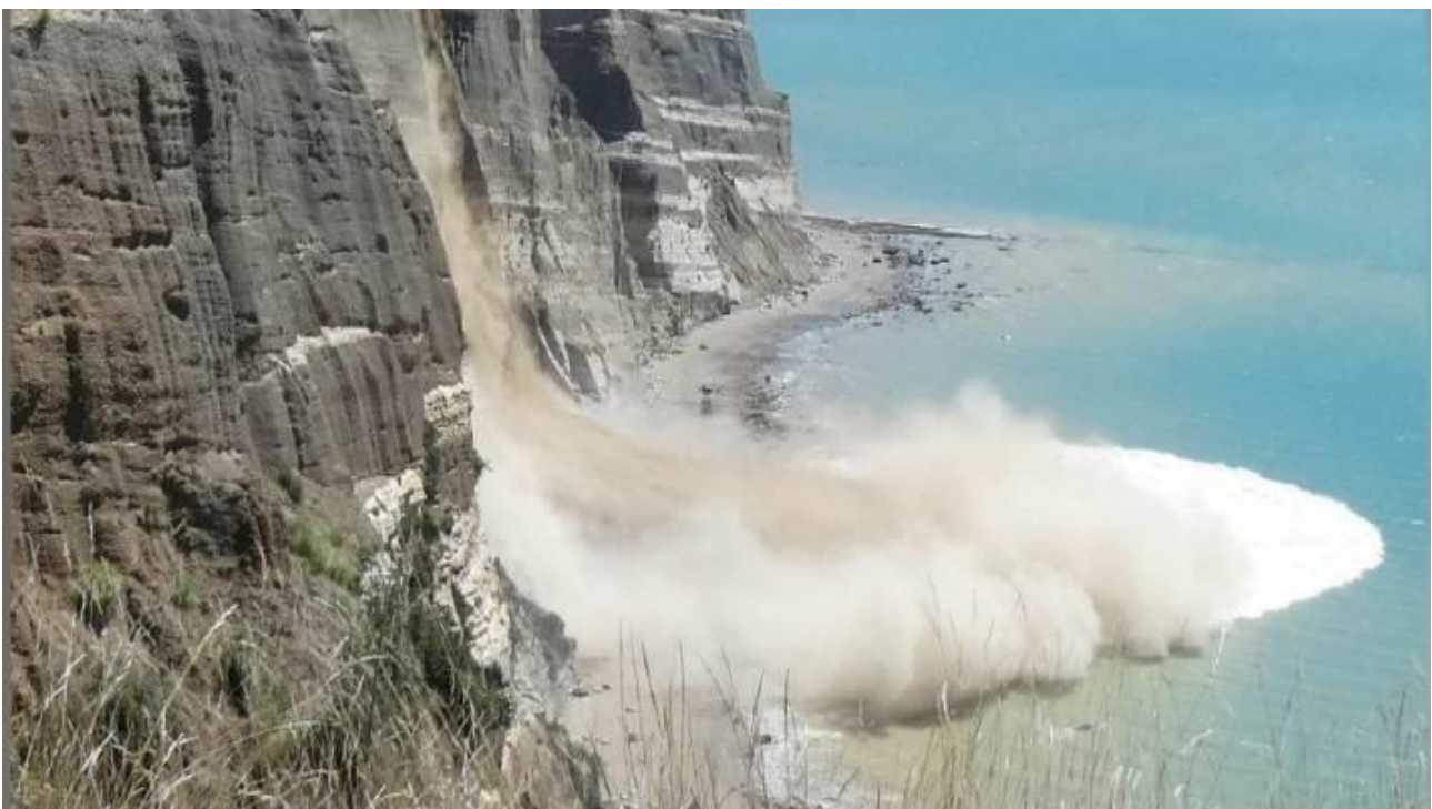
Figure 2: Web Image captures the moment a cliff collapsed at Cape Kidnappers.
