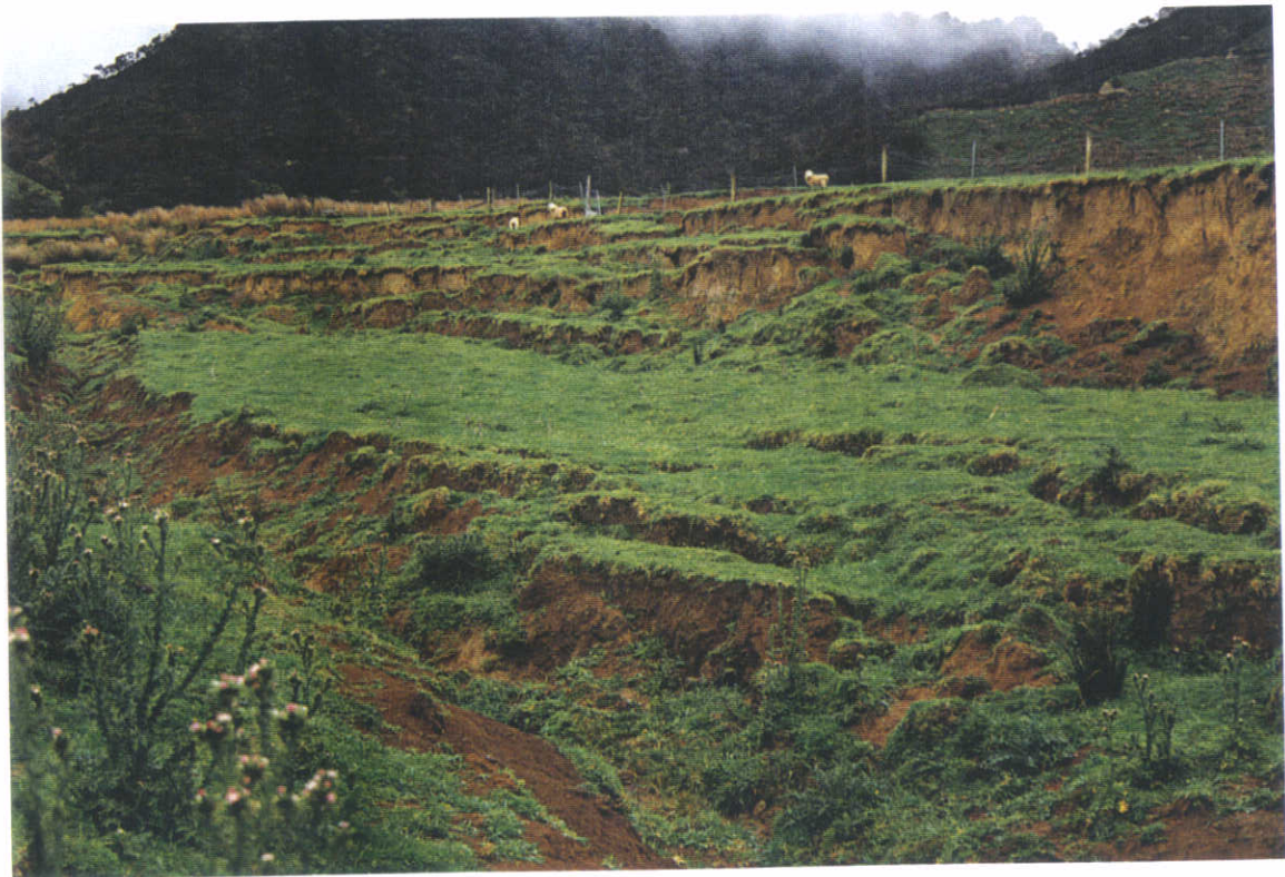
Figure 5 Multiple scarps indicating ongoing slide movement of the ash slope
