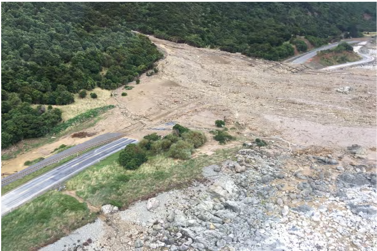
FIGURE 9.1. Damage to Road and Rail as a Result of the Jacobs Ladder Debris Flow, North of Kaikoura, February 2018. (photo supplied by NCTIR)
