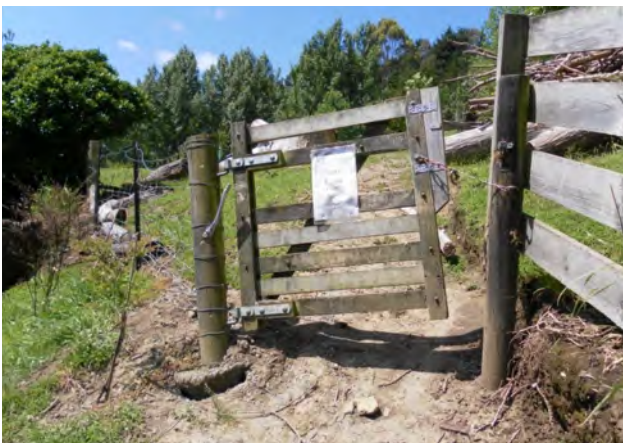
FIGURE 3.3. Displaced gate and fence caused by differential movement within a landslide
