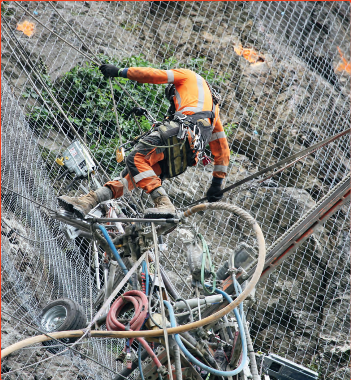
Anchor Installation, Kaikoura Coast, January 2018. Photo courtesy NCTIR
