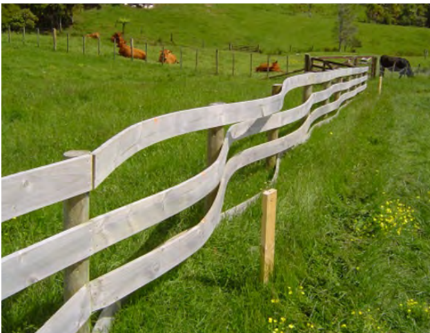
FIGURE 3.4. Displaced fence caused by compressive movement
