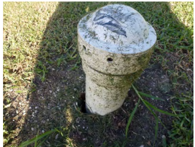
FIGURE 3.6. Ground stretch around a rigid structure (water bore)
