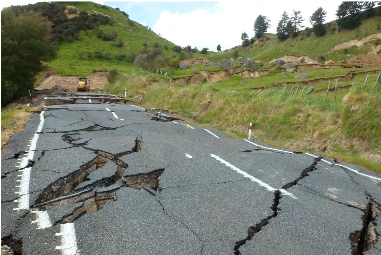
FIGURE 3.10. Widespread cracking in a large translational block slide at Te Oreore (SH4)
