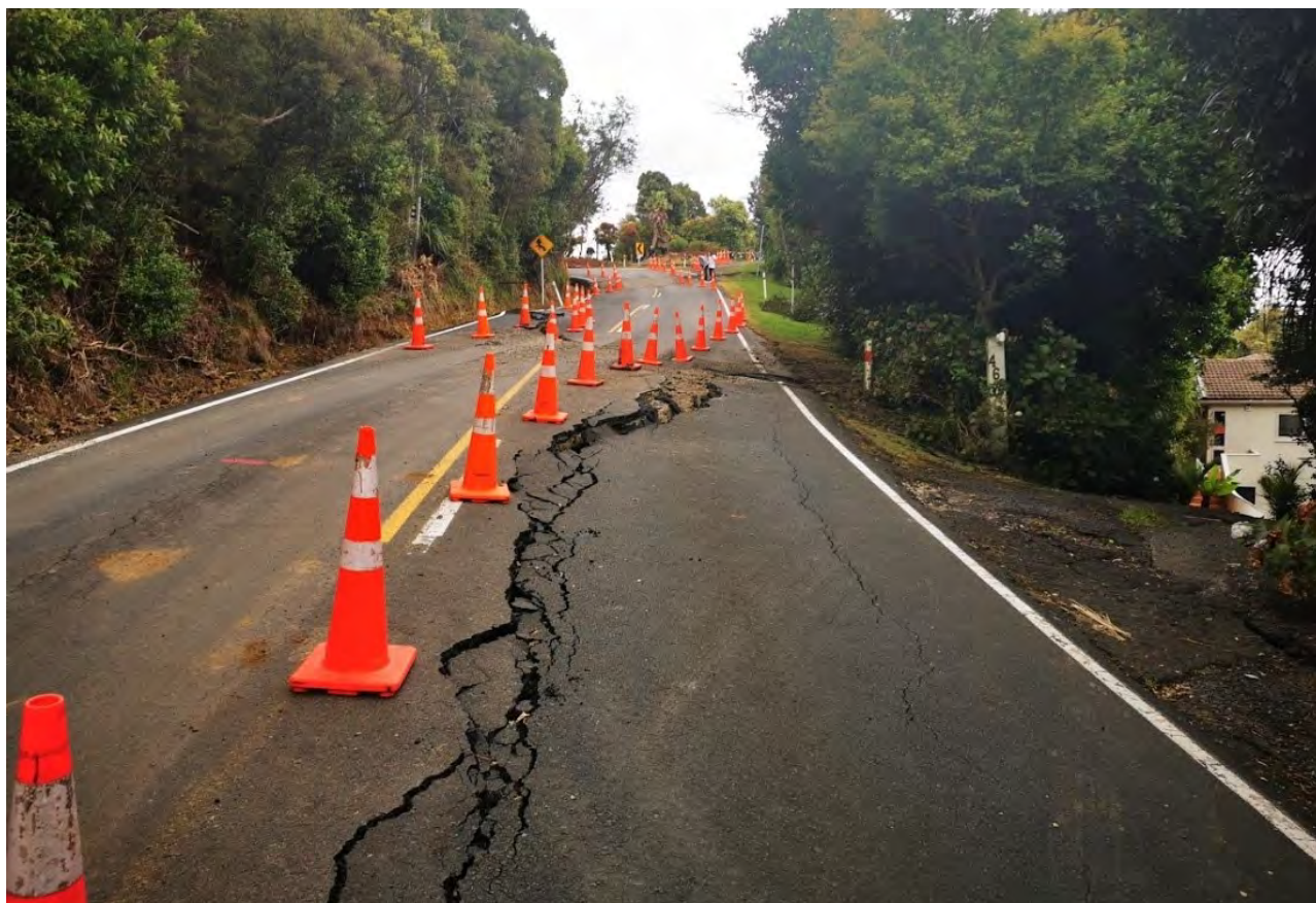
FIGURE 6.8. Example of incipient failure requiring risk assessment to determine immediate, short- and long-term risks. Assessment to consider risk to road users and house resident and maybe other stakeholders (e.g. utility providers). Photo provided by Ross Roberts, Chief Geotechnical Engineer, Auckland Council, 2023.
