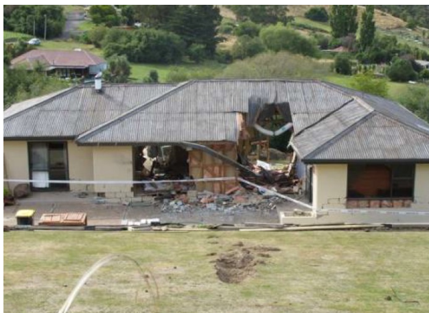
FIGURE 51: Rolling boulder damage to a house in Rāpaki (Dellow et al, 2011).
