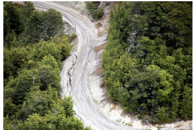
FIGURE 58: Cracks along outboard edge of mountain road above Mount Lyford (Jibson et al., 2018).
