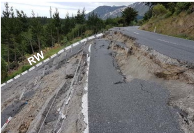
FIGURE 57: Translational failure of fill embankment and gabion retaining wall (RW) north of Kaikōura (Mason et al., 2023).
