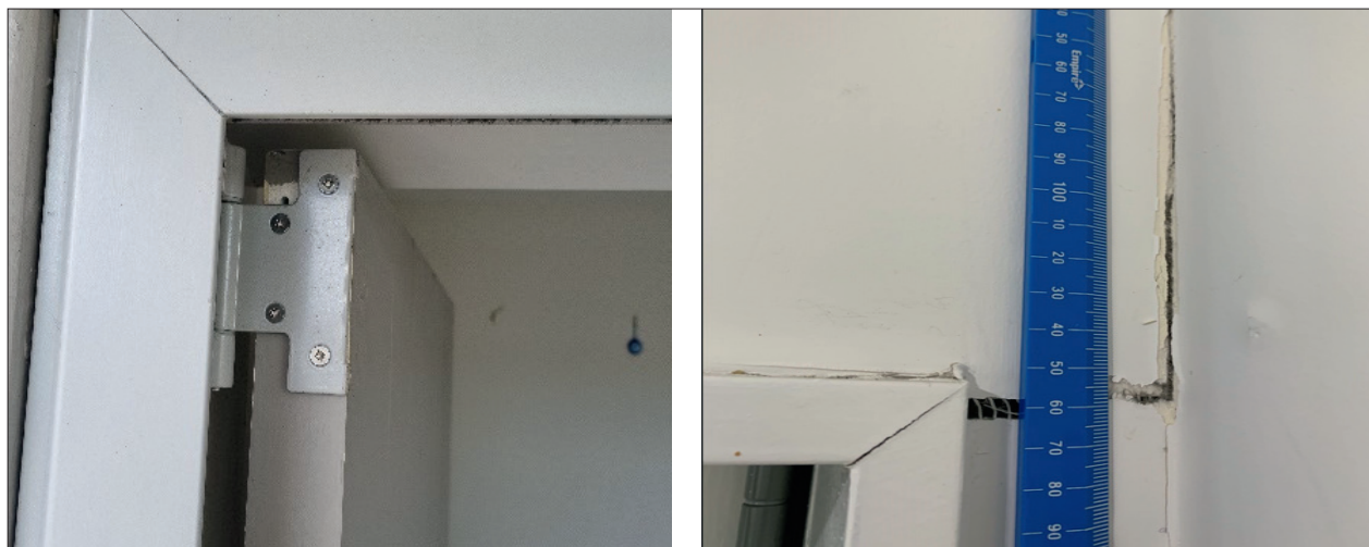
FIGURE 2: (a) Adjusted door hinge and (b) Crack in the corner of door frame, showing clear signs of movement.
