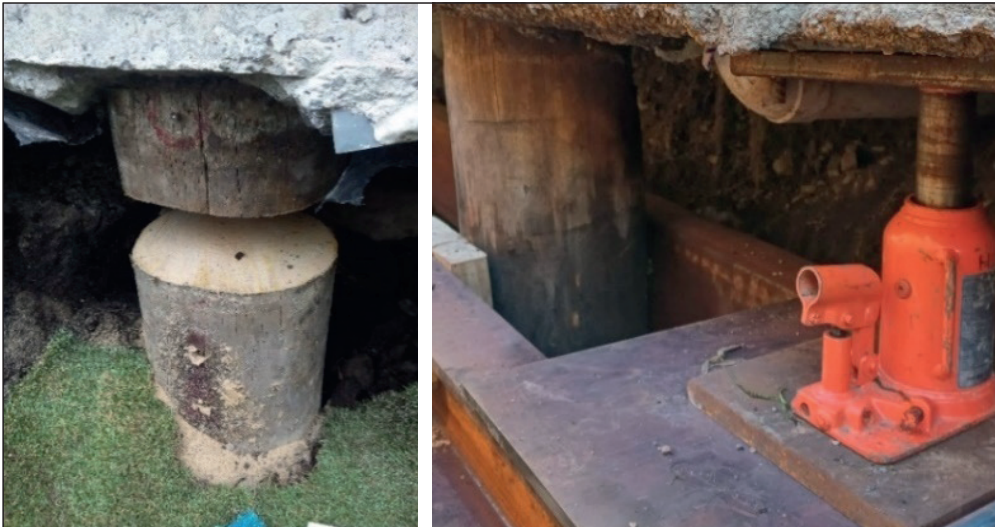
FIGURE 4: (a) Jacks between jacking beam and underside of the rib-raft foundation and (b) Pile Cut
