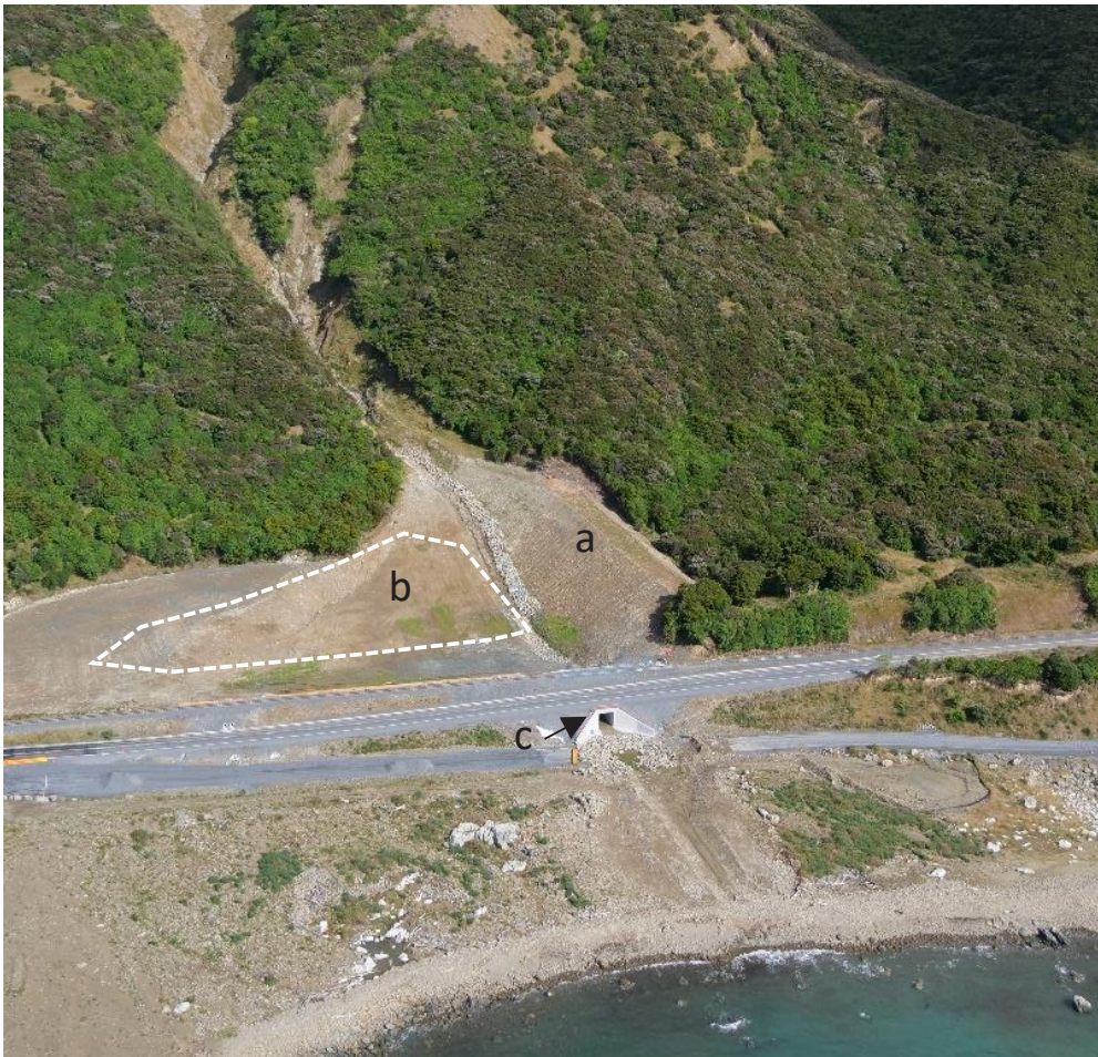
FIGURE 46: Open Control Structures at Jacob's Ladder (a) lateral berm (b) depositional basin (c) large dimension culvert under the transport corridor for conveyance of residual flow. Photo courtesy NCTIR.
