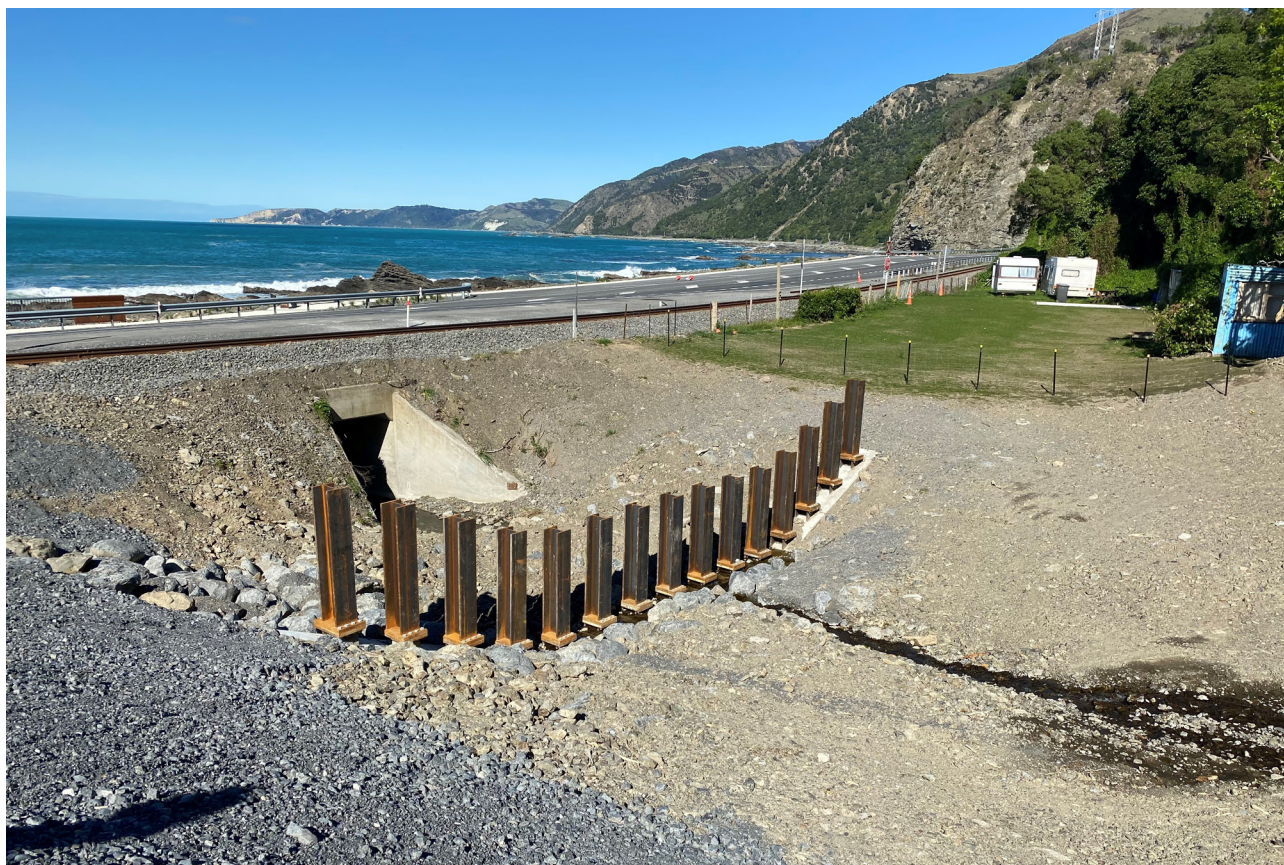
FIGURE 51: Debris Straining Structure, Rosy Morn Stream. Photo courtesy NCTIR
