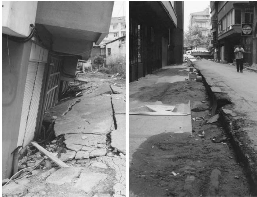
Figure 1: Examples of foundation bearing capacity failures in Adapazari following the Izmit Earthquake, Turkey 1999 (Bakir, et al., 2005).
