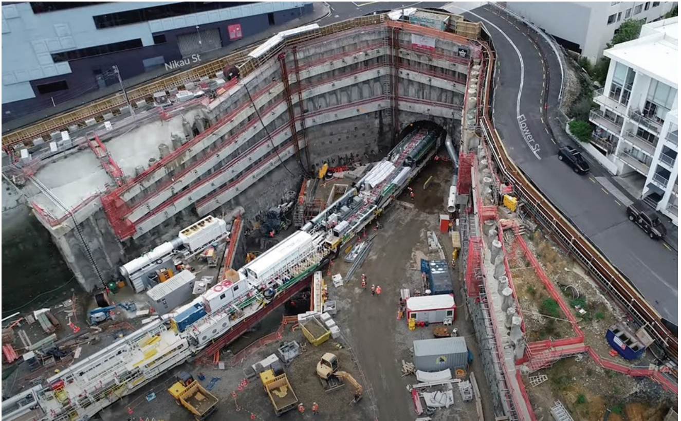
FIGURE 1: Mt Eden tunnel portal temporary retention structure with TBM Dame Whina Cooper in foreground.
