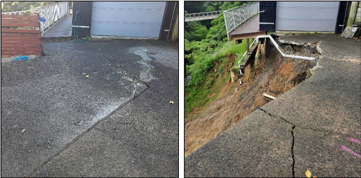
Figure 2: Regression Landslide Crest Observed (two photos taken five months apart)
