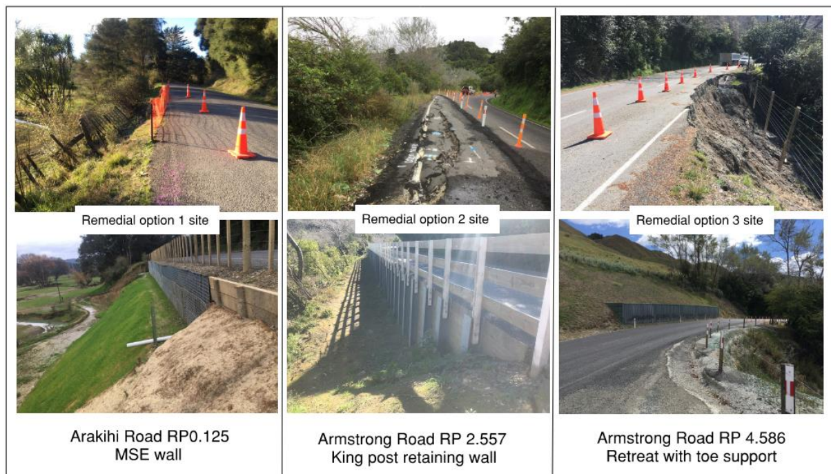
Figure 5: Examples showing the initial storm damage and final constructed design for each remedial option.
