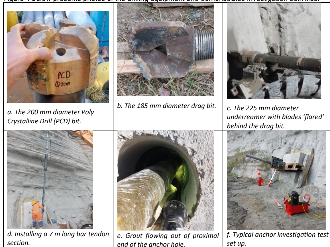
Figure 4: Construction and testing photos from investigation trial.
